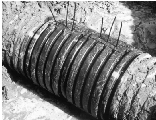
Figure 3 Split Band Installation
